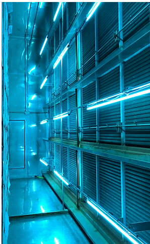
Fresh-Aire UV Air Handler Disinfection: Installed inside the AHU, the Fresh-Aire UV TRS system disinfects air handler and equipment.
